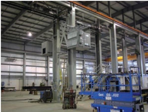
**Smog-Hog systems are arranged in a racetrack configuration.**
